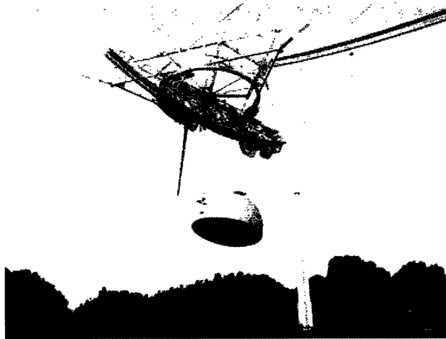
Figure 14. On May 16, 1996, the new Gregorian dome was lifted to the platform.
